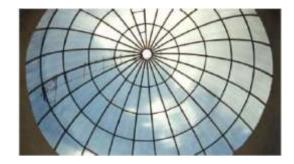
Figure 17. Day lighting with poly carbonated sheets
